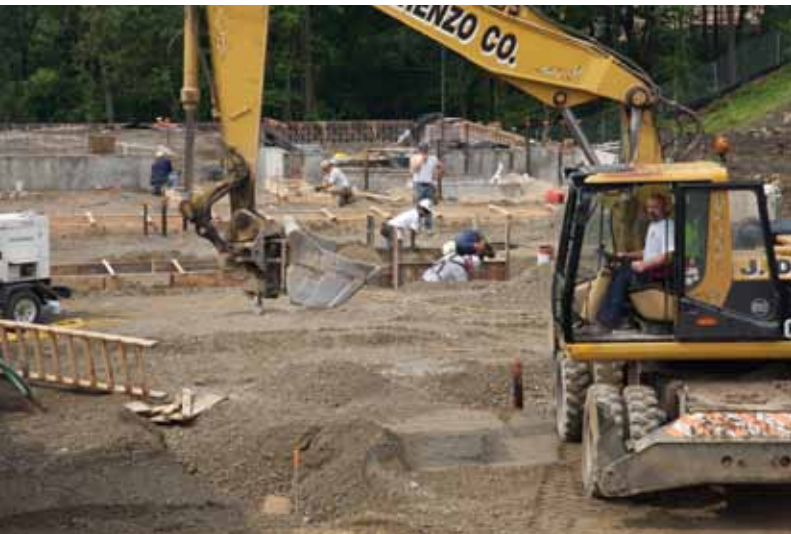
Work began as soon as the celebration was over.
